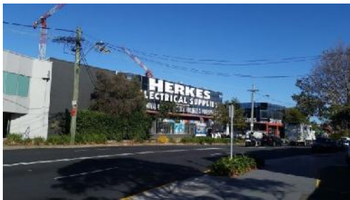
Figure 9: Looking south-west along Bourke Street towards subject site and adjoining site at 890-898 Bourke Street
