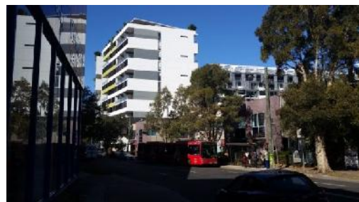
Figure 6: Looking south-east towards site from O'Dea Avenue.
